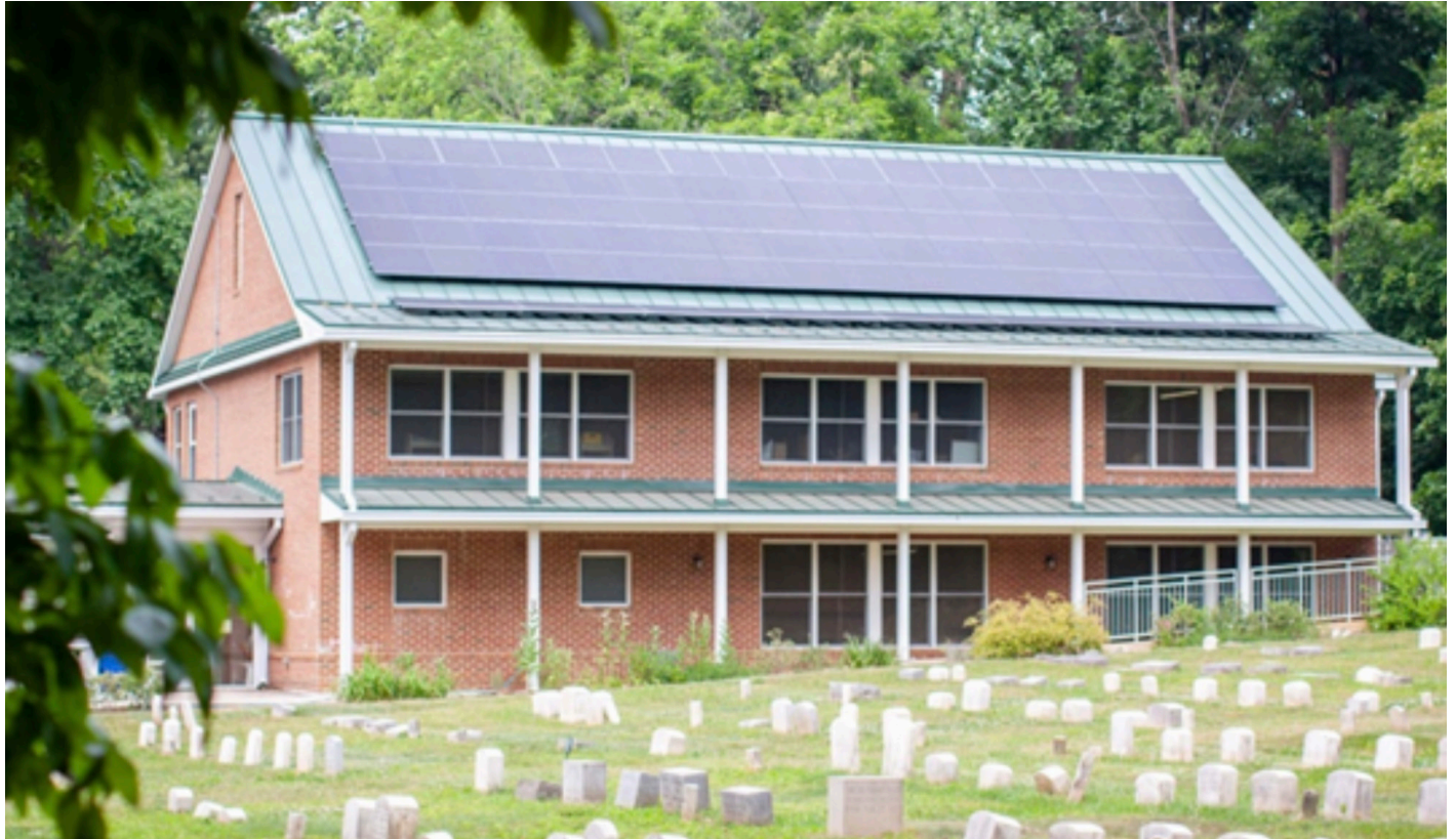
New Solar Panels at Sandy Spring Friends Meeting Community House
