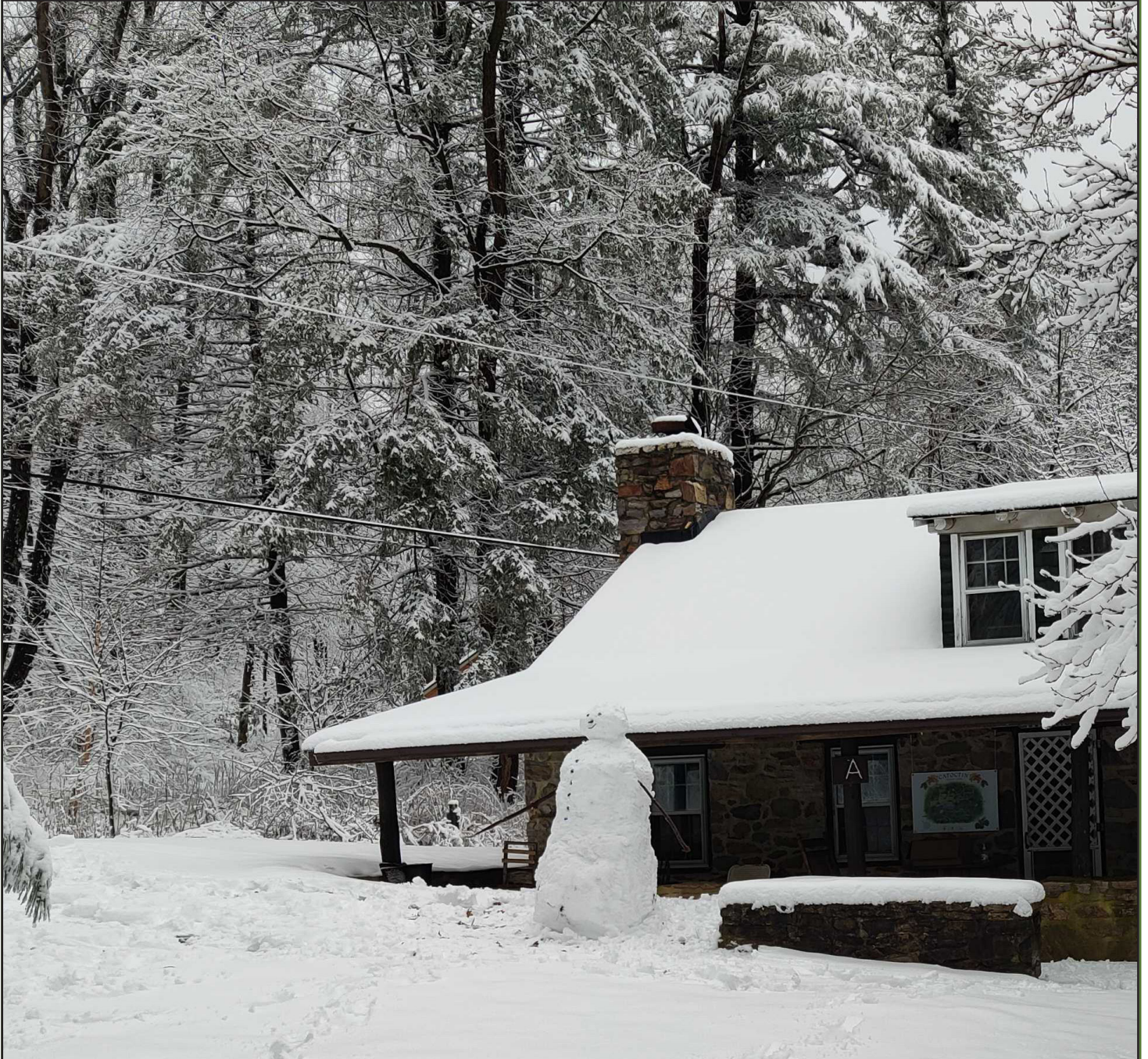
Rolling Ridge progress 2024
