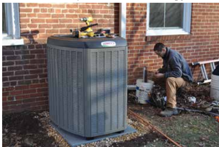
Valley’s New Heat Exchanger
