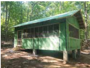
Cabins almost completed
