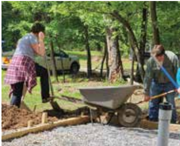
Volunteers hard at work on the shower house porch
